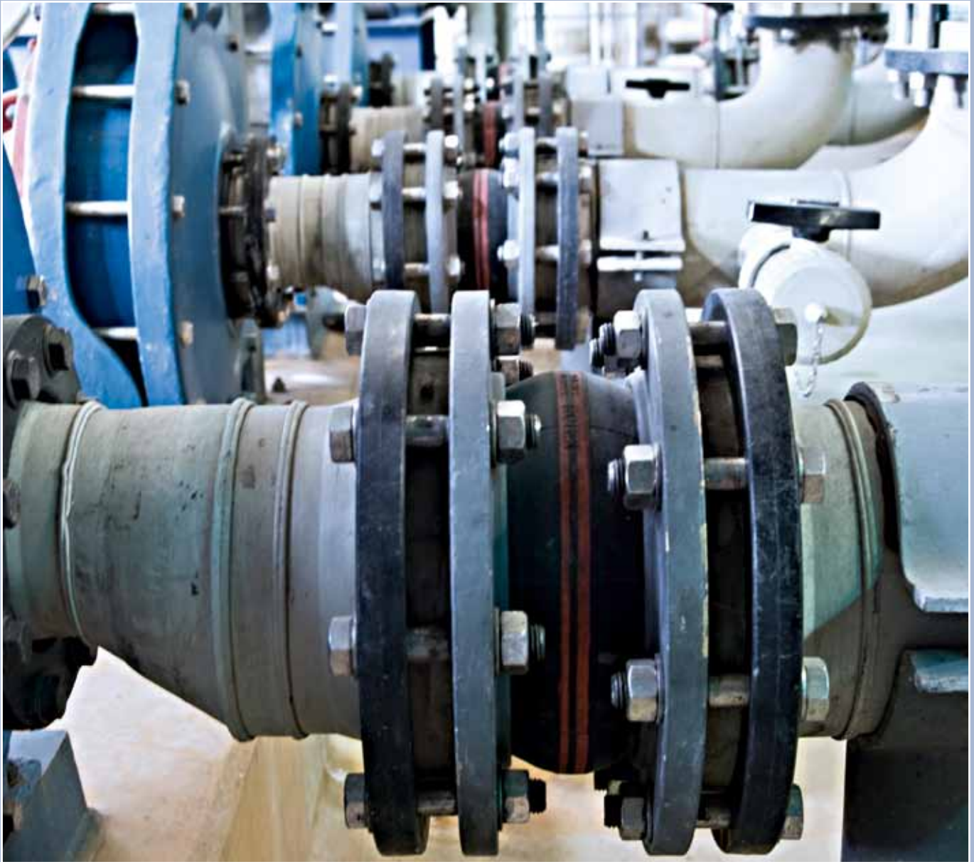
Universal expansion joint, type D100A on the suction side of quenching water pumps in a waste incineration plant NB 150, 16 bar
