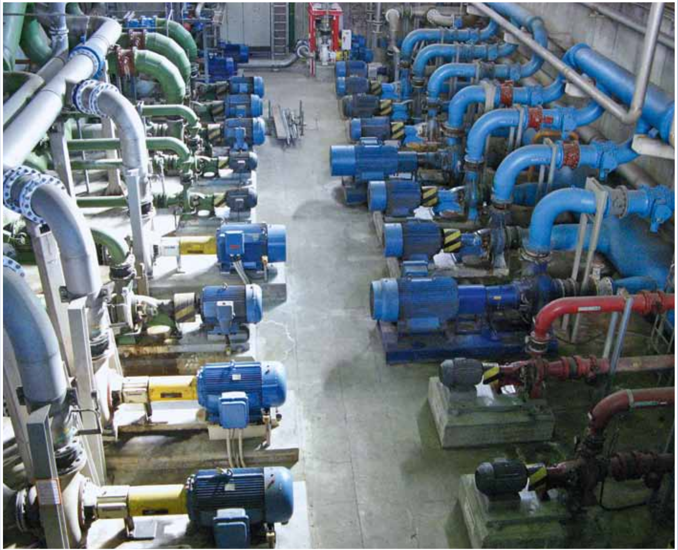
Universal expansion joint, type U110A on the supply pumps in a paper mill DN80 – DN350, 10 bar
