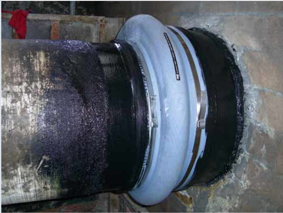
Wall seal, type W111SS, on a cooling water pipe in a nuclear power plant NB 700 / NB 600, 0.25 bar from outside
