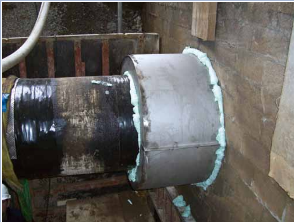
... after installation of a ground protective cover
